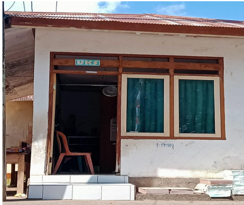
Ruang UKS MTs Abul Abbas
