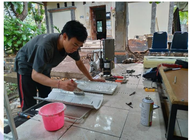
Gambar 2. Tahap pengecatan kasing unit outdoor
