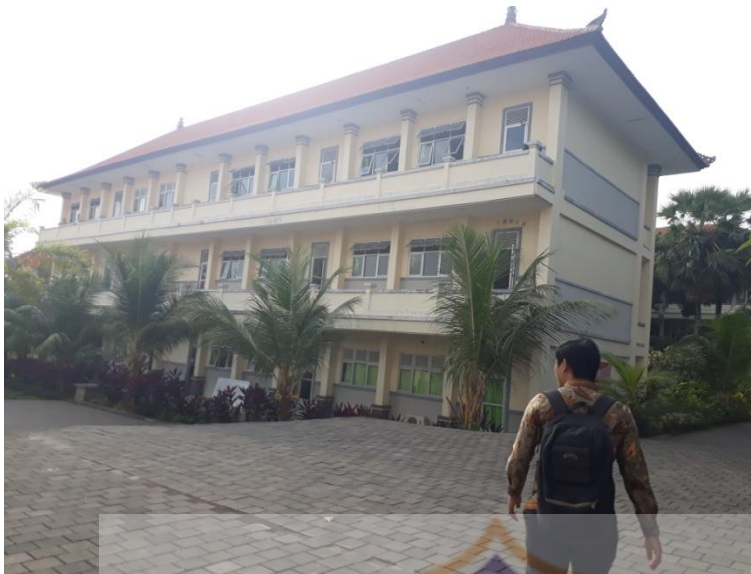
The classroom of architect engineering department students is in the third floor
