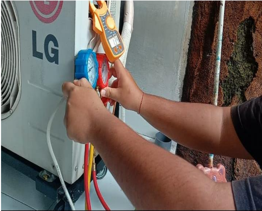
Penambahan refrigeran AC
